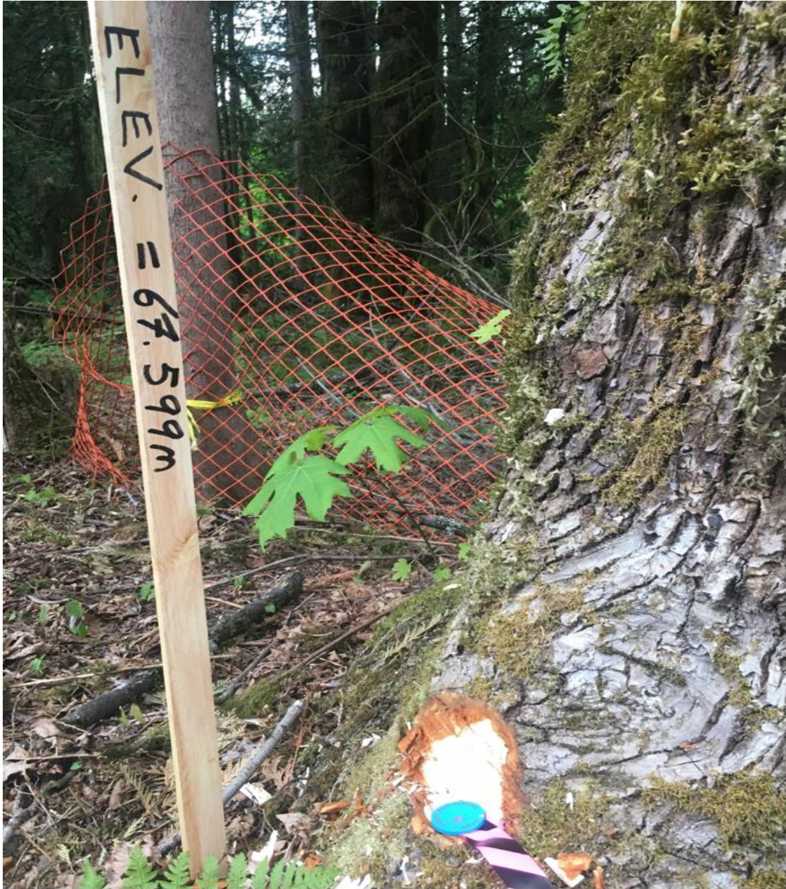
Figure 6 - Site Surveying (FVRD, 2019)
