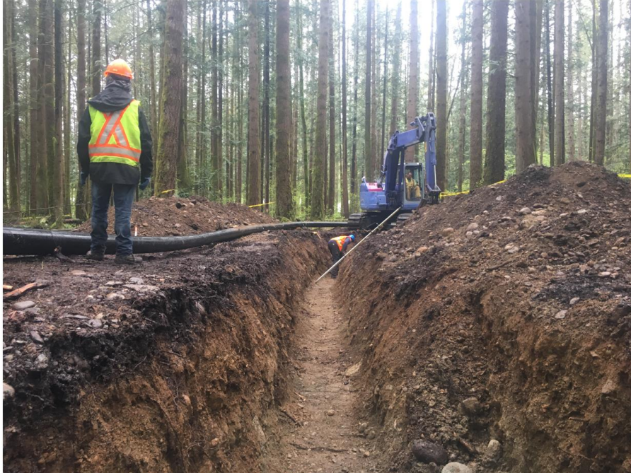
Figure 9 – Trenching for Forcemain to Site (FVRD, 2019)
