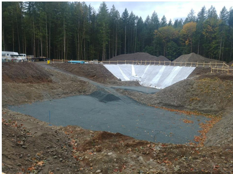
Figure 7 - Site Excavation to Subgrade (Urban Systems, 2019)
