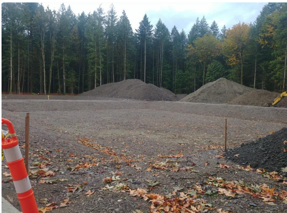
Figure 8 - RIB Excavation (FVRD, 2019)
