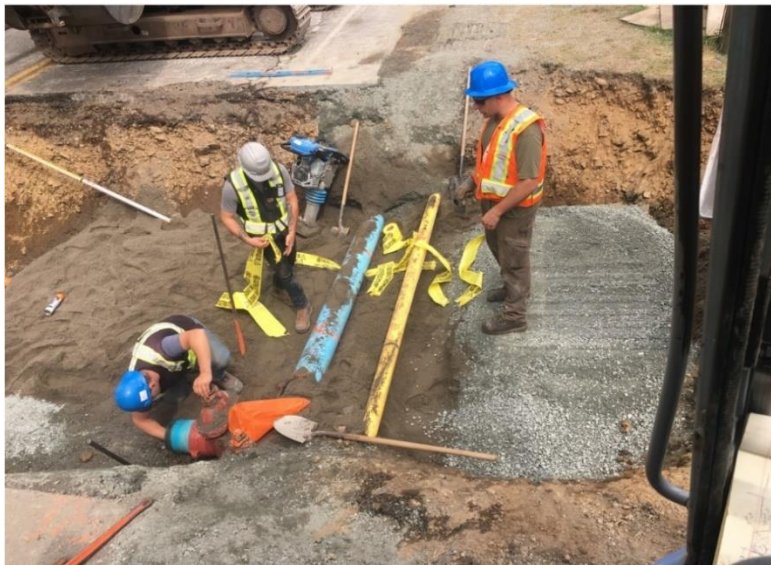
Figure 5 - Gas/Electrical/Communications Conduits for Road Crossing (FVRD, 2019)
